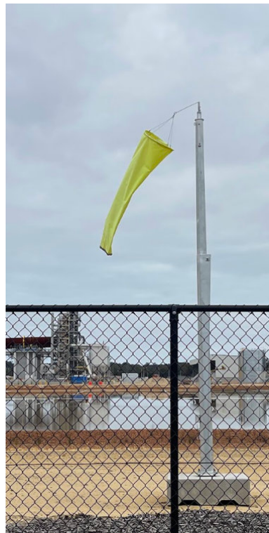
Kemerton - Lithium processing plant - Bunbury, WA
