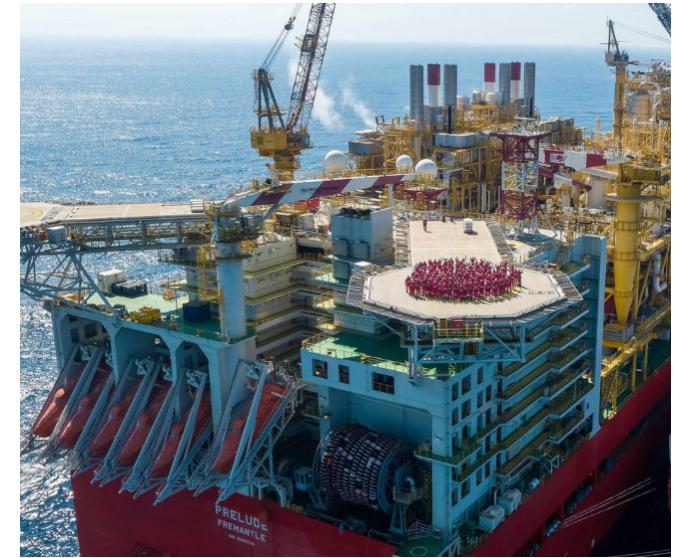
Proud supplier to Shell's Prelude FPSO: Source Shell
