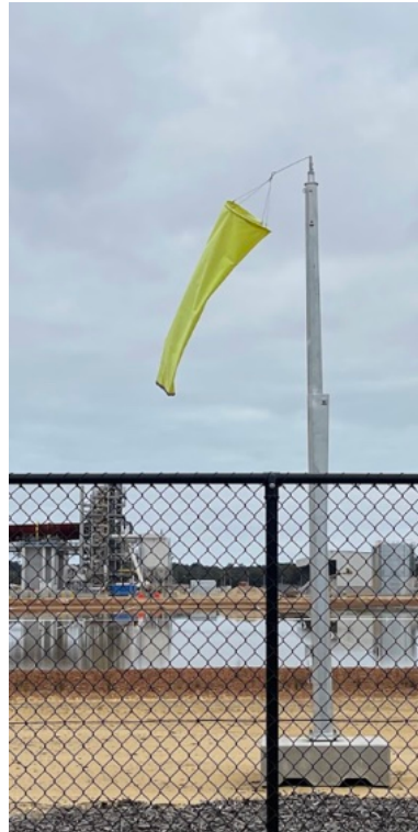
Kemerton - Lithium processing plant - Bunbury, WA
