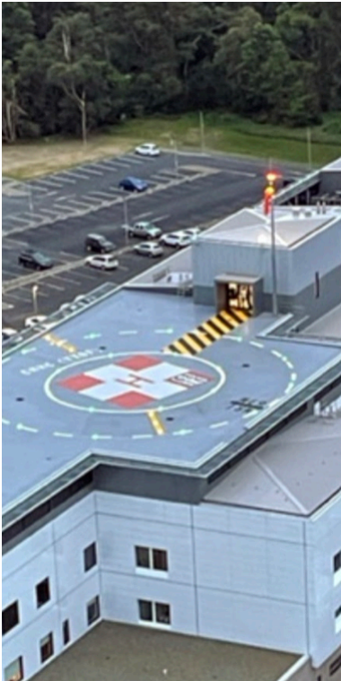
NSW Health - retro fit HLS IWDI Windsack assembly - North Coast, NSW
