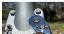
Step 1: Loosen bracket bolt
