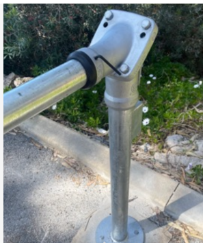
Base-mounted swivelling joint
