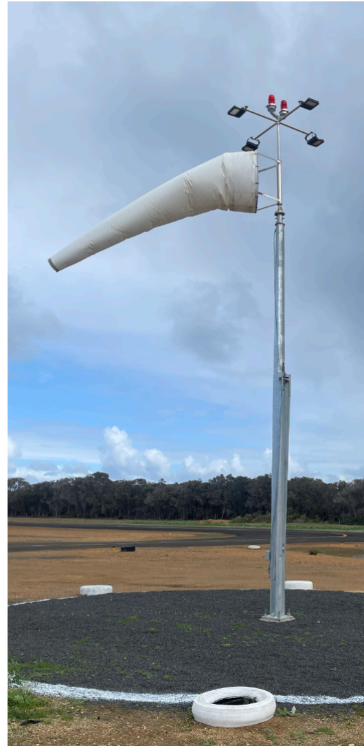
Augusta Airport, WA - Indicative Installation. IWDI with LEDs and Obstruction Lights mounted on fully SS Dual 900m Ø Windsock Frame with CASA Aviation Grade Windsock. IWDI is mounted on 6m Extra Heavy Duty Counter Weighted Galvanised Pole
