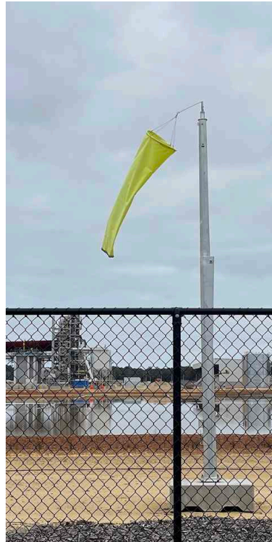
Kemerton - Lithium processing plant - Bunbury, WA
