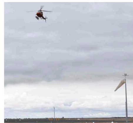
CASA compliant Illuminated Wind Direction Indicators (IWDI) used for night time operations at airports and helicopter landing sites
