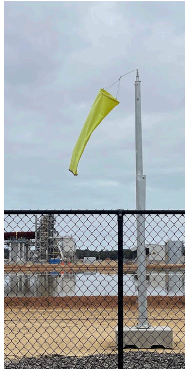
Kemerton - Lithium processing plant - Bunbury, WA
