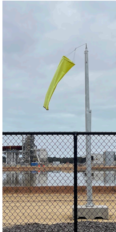
Kemerton - Lithium processing plant - Bunbury, WA
