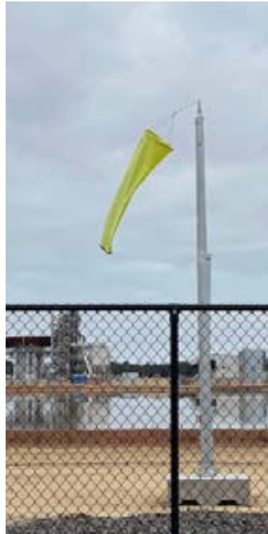
Kemerton - Lithium processing plant - Bunbury, WA
