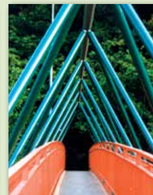
▲ Footbridge in San Sebastian, Spain.
