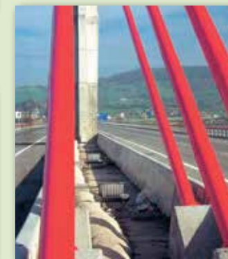
▼ PPA 571 coated suspension cable covers after ten years in Spain.
