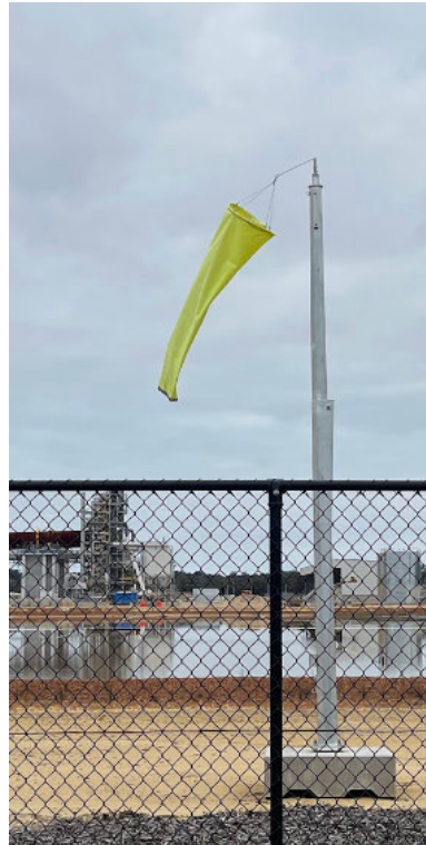
Kemerton - Lithium processing plant - Bunbury, WA
