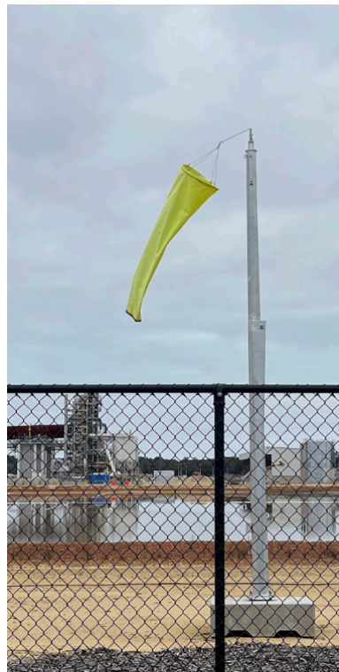
Kemerton - Lithium processing plant - Bunbury, WA
