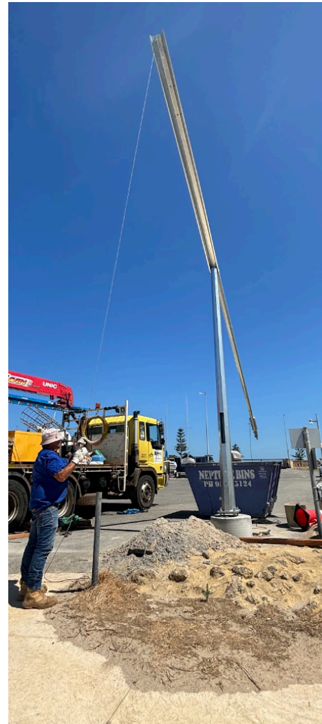
The design of the mid hinging, counterweighted pole eliminates the need for an elevated work platform, with all work able to be carried out at ground level
